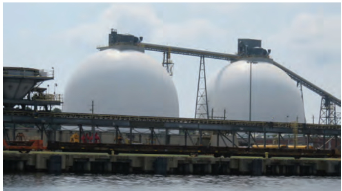
Photo: RCC, Alexandra Wisner, 2018, Enviva Wilmington, NC Port storage facility 9
