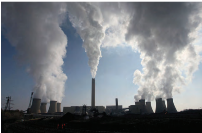
Photo: Andrew Whale, 2011, Drax Power Station 4
