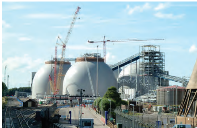
Photo: Chris Allen, 2013, Drax Biomass Storage 3
